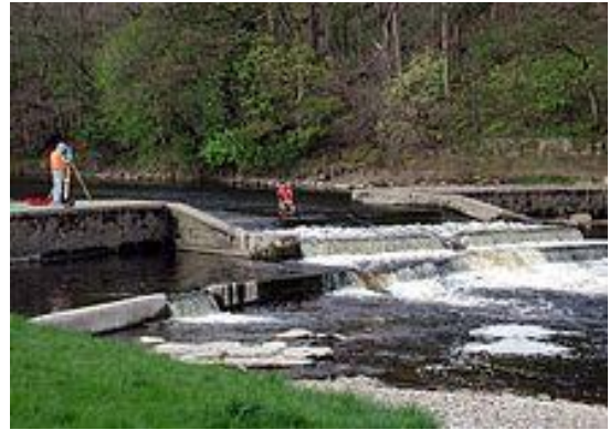
Weir at Low Mill
